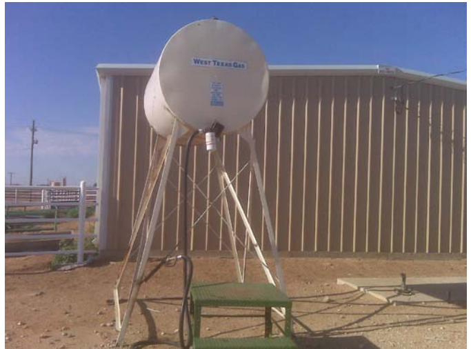
500-Gallon Rodeo Diesel Tank (T2)
