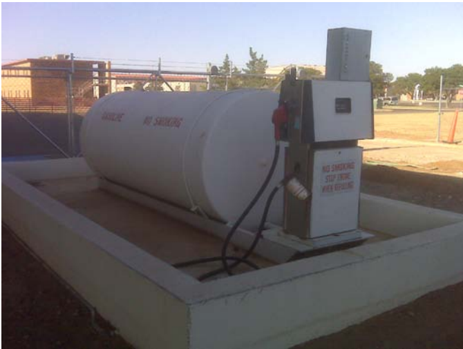
1,020-Gallon Warehouse Gasoline Tank (T1)
