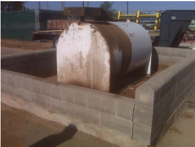
500-Gallon Auto/Diesel Used Oil Tank (T3)
