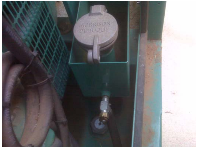
200-Gallon Fine Arts Emergency Generator Belly Tank (EG)
